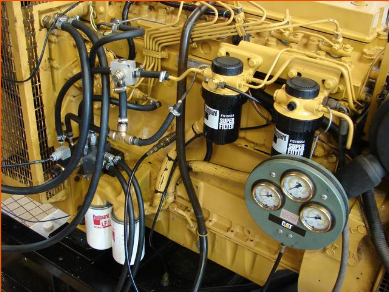
Modification circuit gasoil
